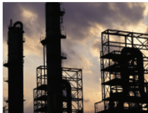
indoor/outdoor transitional links at electrical substations
